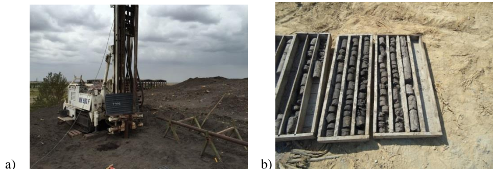
Fig. 5. (a) Drilling plant; (b) Stratigraphic column - obtained from core drilling
